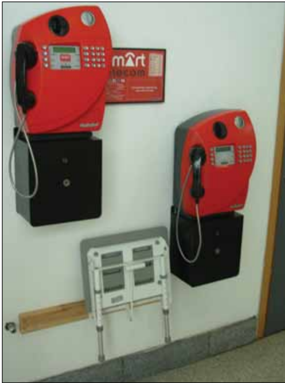
Image 6.4. Example of two payphones fitted at different heights.
